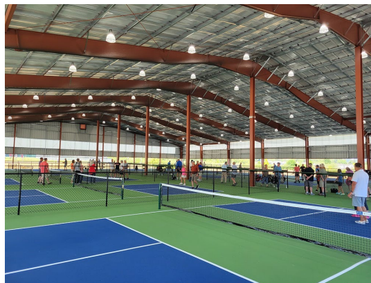
Blackburn Pickleball Pavilion Mount Vernon, WA
